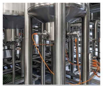
With IO-Link sensors for temperature, turbidity, conductivity, level, flow and pressure, Anderson-Negele can offer almost all measuring ranges from a single source. Thanks to Flex-Hybrid technology, sensors can be operated in digital and analog mode in parallel (IO-Link and 4...20 mA).
