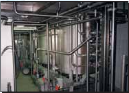
Leveltransmitters on CIP tanks
