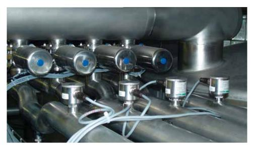
FLOW MEASUREMENT OF DEMINERALIZED WATER
